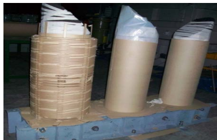
Figure 4.9(a): Core coil assembly in progress
